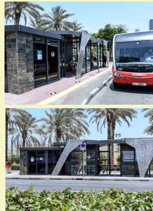
Figure 5: New bus shelters
